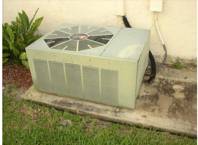
metal "fins" that allow the coils more surface area to exchange heat. Follow these tips when cleaning the exterior condenser unit and its inner components -- after turning off power to the unit!
